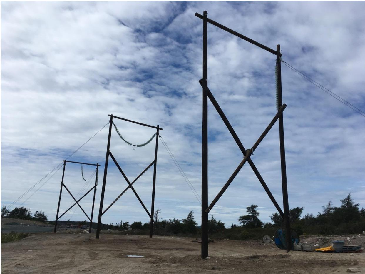
Figure 2 - Completed Wood Pole ERS at SOP
