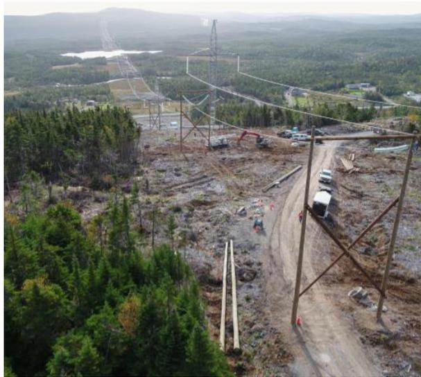
Figure 5: Wooden Pole Solution Used in 2018 Mock Exercise
