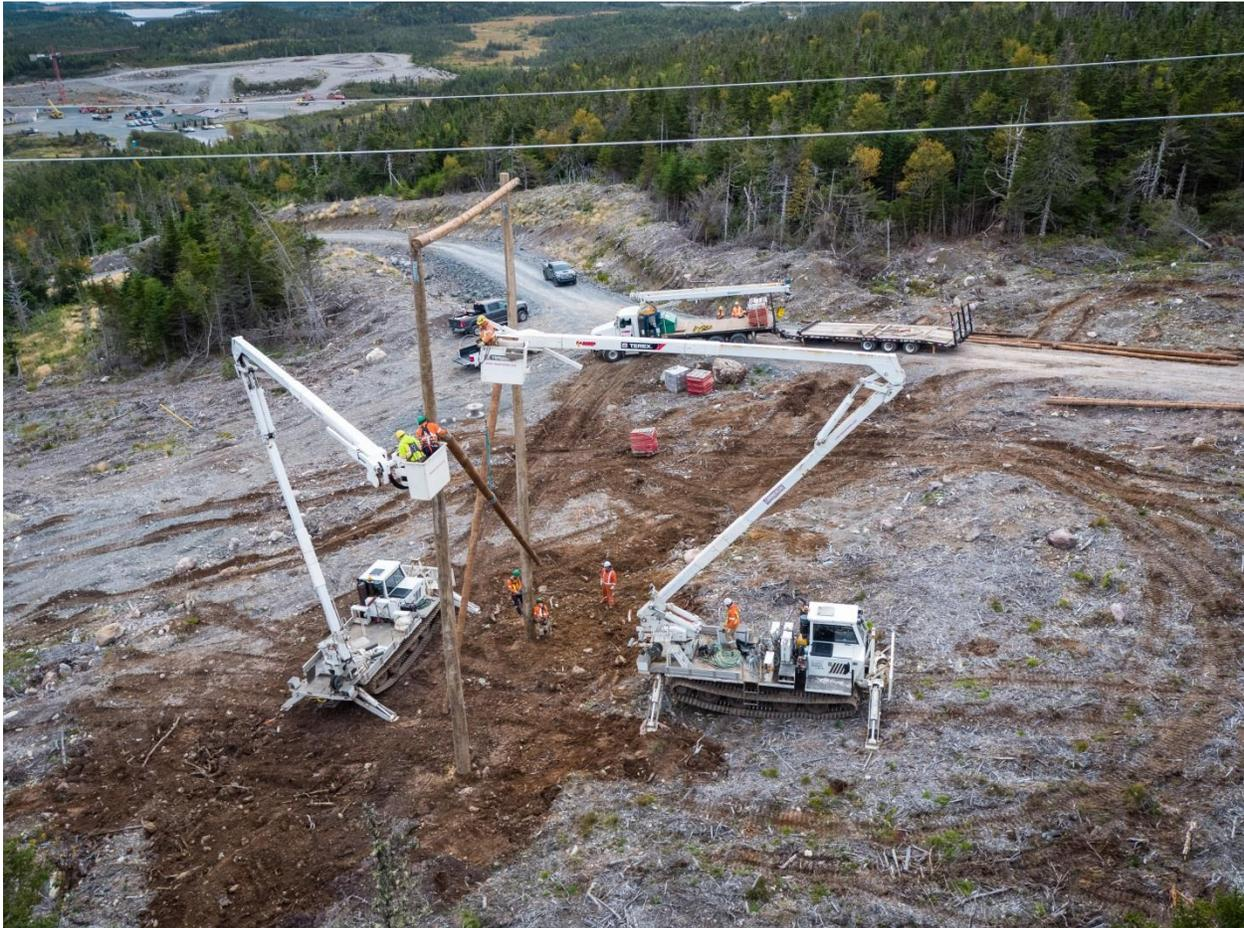
Figure 5 - Construction of Tangent ERS.
