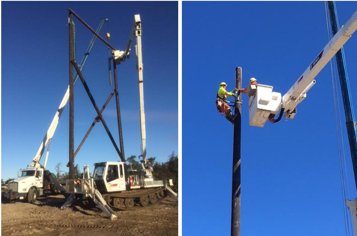
Figure 1- Wood Pole ERS Construction at SOP
